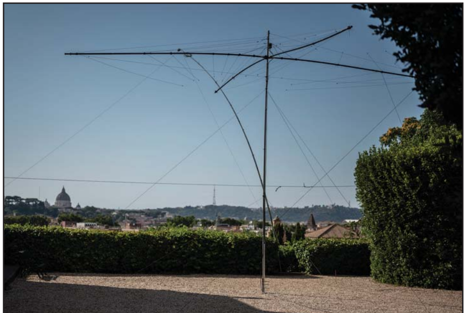
Photo J. The 5-band Spiderbeam Yagi on the terrazza of Magistral Villa (Photo by IZ4AKS)
