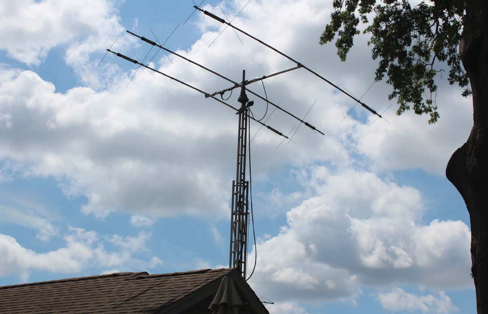
Photo A. My 40-foot tower and 3-element beam
