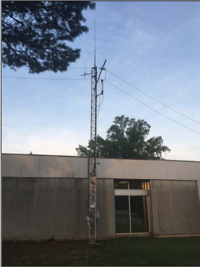
Photo H. Exterior shot of the NWS Memphis office. Note the tower with amateur radio antennas supporting SKYWARN®.
